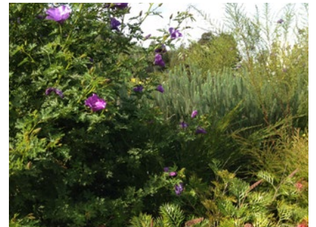
The Burnley Campus Green Roof which demonstrates our research outcomes.
