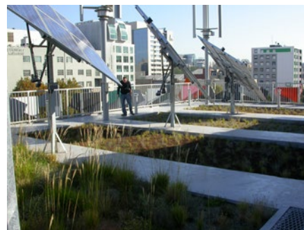
The Pixel Building Green Roof in Carlton used green roof plant palettes and substrates based on our research. It was designed to reflect the pre-European vegetation at the site and provide biodiversity habitat.
