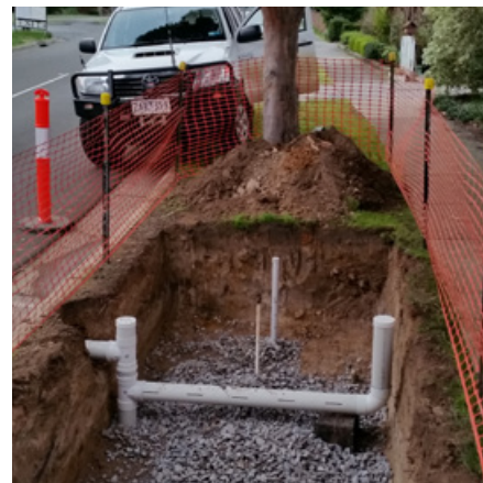
Constructing a system to irrigate street trees with stormwater generated by roads.
