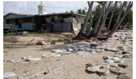
Coastal erosion, Lifuka, Ha'apai Tong.
