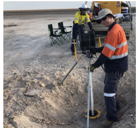
CSIRO colleagues installing a fibre-optic cable in a bore drilled by Geoscience Australia in the Northern Territory in December 2020. The cable will allow measurements of temperature and thermal conductivity to 500m depth to investigate crustal heat, aquifer properties and atmospheric temperature changes.
