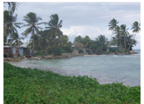
Ad hoc sea walls, Majuro, Marshall Islands.
