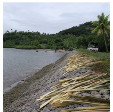
Rock revetment to slow coastal erosion and flooding, Karoko, Fiji.
